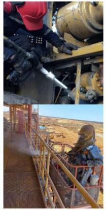
Wet blasting is especially effective for dust control and environmental compliance. By ensuring proper surface preparation, abrasive blasting maintains equipment integrity, supporting operational efficiency and safety.
